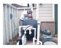
Step 4. Remove existing sand media from filter tank. A heavy-duty shop vac comes in handy for this step. Otherwise remove by hand, or if filter is equipped with a sand drain plug, remove plug and washout sand through the drain.
