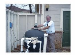
Step 2. Release air pressure from filter tank. Carefully remove filter tank cover and move distributor for access to media bed. (Consult filter manufacturer's manual for specific directions concerning filter piping)
