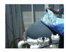
Step 6. Fill filter tank with the required amount of Zeobrite Filter Media. (Note: Zeobrite weighs 50% less than sand per cubic foot, therefore, it requires 50% less weight of Zeobrite versus sand.) See the Media Requirement Chart below.
