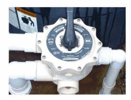
Step 8. Turn multi-port valve to the backwash position. Start filter pump and backwash the media until the water in the site glass is clear (usually 2-3 minutes). Turn-off filter pump and proceed to Step 9
